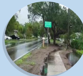
Flooding and drainage issues
