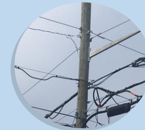
Street Lights and overhead utilities
