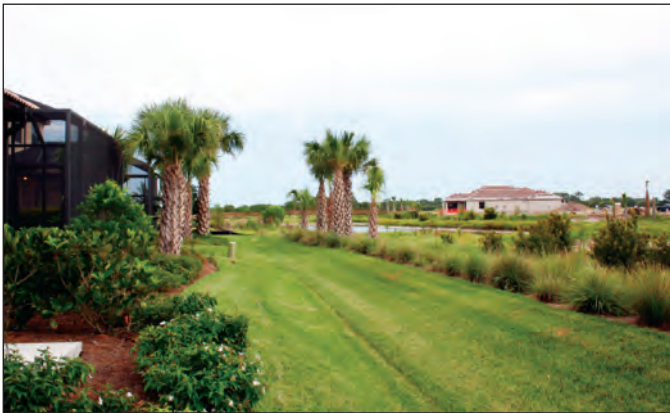
Swales encourage stormwater to soak into the ground.
