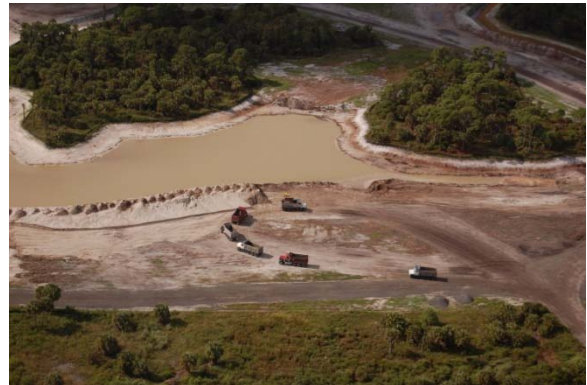
Removal of fill at Winding Waters
