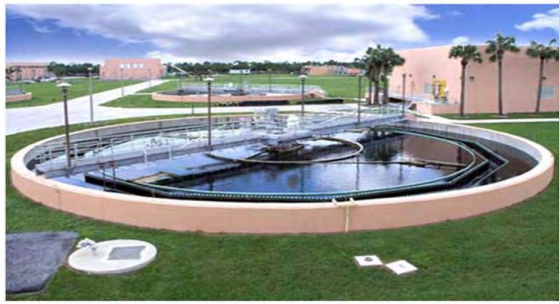
Southern Regional Water Reclamation Facility
