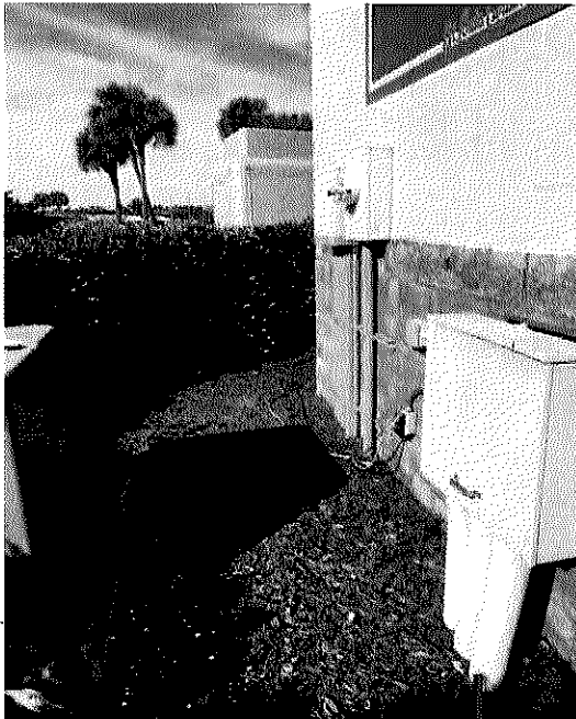
Conduit coming through the pull box with available space, road and pull FOC
