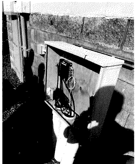
Conduit coming through the pull box with available space, road and pull FOC
