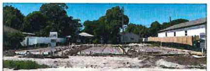
Three CLT homes in progress on North E Street.
