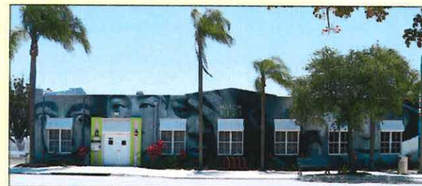
HATCH 1121 has become the location that connects the community through culture and the arts, located in the Lake Worth Beach Arts Overlay District and operated by LULA Lake Worth Arts. Renovations for the center were funded through a cultural facilities grant awarded by the State of Florida's Department of Cultural Affairs.
