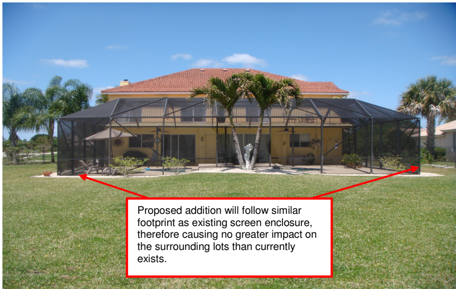
Rear Yard Looking Toward
