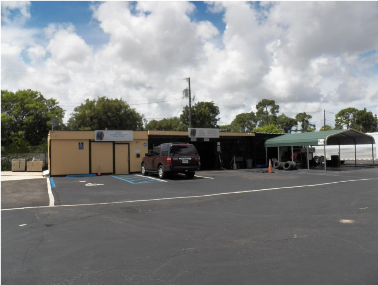
View looking south at Building C
